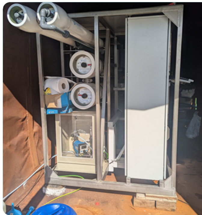
ASTRO leachate treatment system with ZwitterCo Elevation High Pressure RO Membranes
